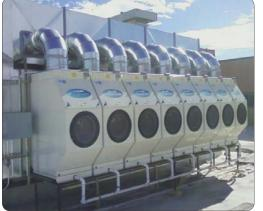
The Coolerado air conditioner uses 90 percent less energy compared to typical air conditioners — and it reduced our carbon footprint by 88 percent per ton of cooling, according to Troy Jensen, Intermountain's energy efficiency manager. The units also have no mechanical parts other than the fan, which will result in significant maintenance cost savings.
